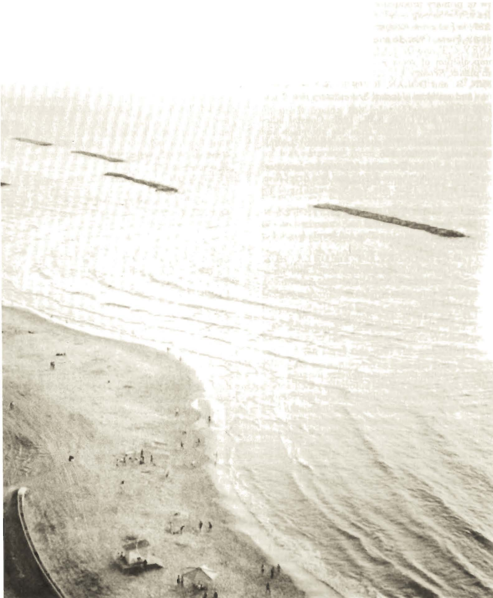
PHOTO43. Longshore of parallel waters at Tel Aviv, with Jaffa in distance. The refracted and intersecting wave patterns favor sand accretion, creating miniature tombolos, and increase effective length of coastline (Photograph by R. W. Fairbridge, 18 Oct., 1980.)
