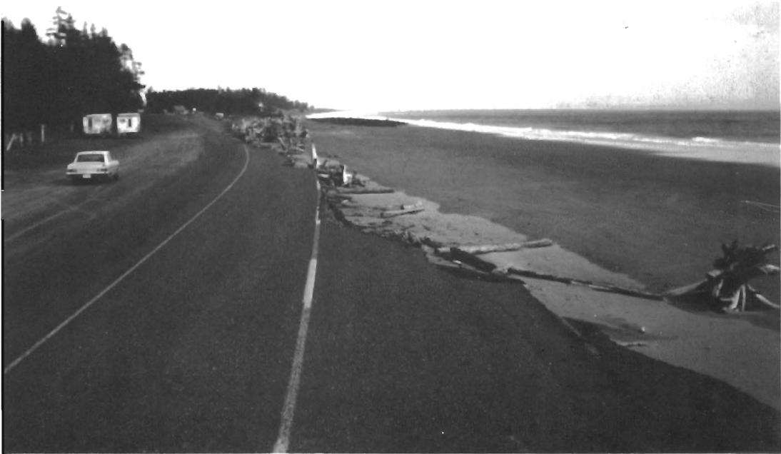
Figure 7. A 1976 view to the east of the old coastal highway eroding away.
