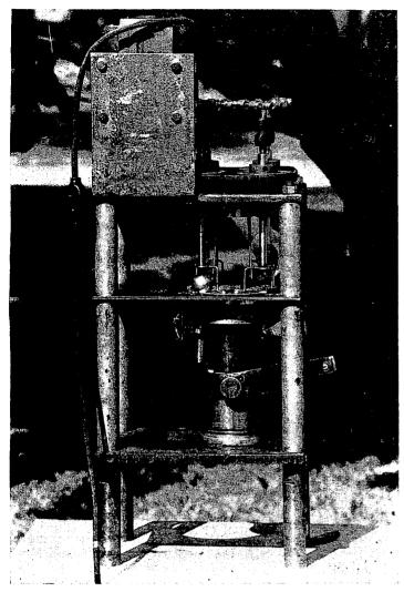
Fig. 1. A multiple cutter machine designed for deseeding muscadine grapes.
