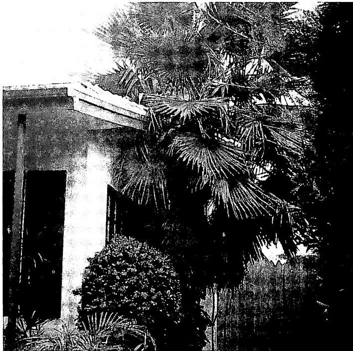
Fig. 3 A stray Mexican Washington Palm that sprang up in an adobe planter against a home on San Marino Island, Miami Beach, putting pressure on the roof. (Photo by Julia Morton)
