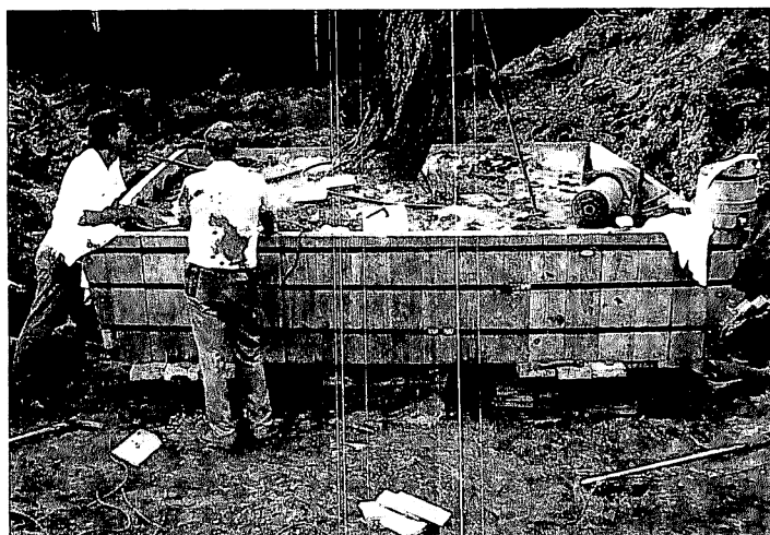
Fig. 2. The bottom planks are being installed from two opposite sides leaving only a four foot wide section of soil in the middle to be removed. The soil has been removed in preparation for placing one plank on each side of the remaining soil.
