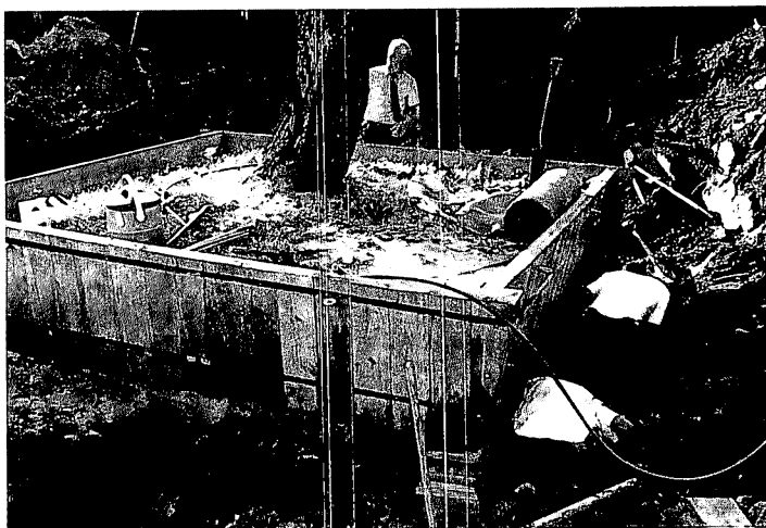
Fig. 1. The sides of the box have been bolted together and strapped securely in place. The first bottom plank is in place.
