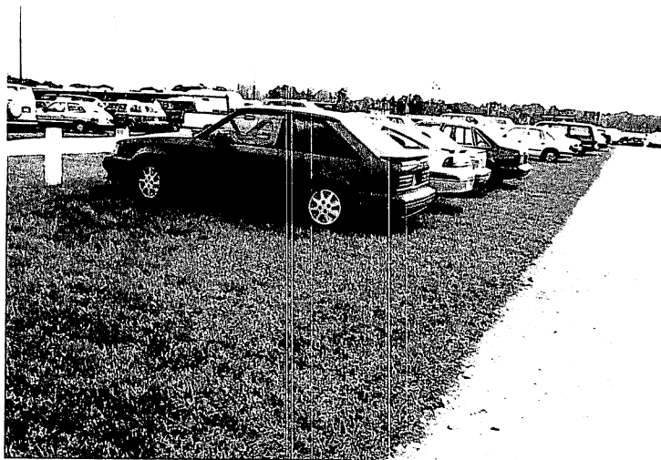
Fig. 2. Parking spaces at Big Top Flea Market are covered by irrigated, 'Argentine' bahiagrass, on sand, while driveway aisles are composed of a pervious, compacted, recycled concrete aggregate underlaid by geotextile fabric.
