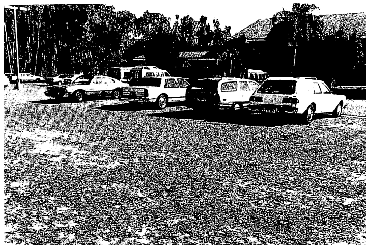
Fig. 3. Turfgrass parking area, Worship Center Baptist Church, Plantation, Florida. This 100% turfgrass area consists of 150 mm compacted base overlaid by 50 mm sand. Although planted to a seed mixture, only 'Argentine' bahiagrass predominates. Weeds are absent.
