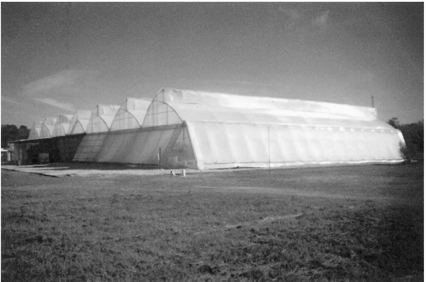
Fig. 1. Passively ventilated, high-roof greenhouse with double layer polyethylene roof and insect screens (Protected Agriculture Project, Gainesville, Fla.).
