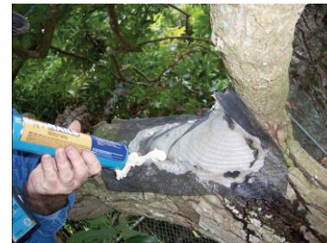
Fig. 7. Adhering window screening over cured expanding foam.
