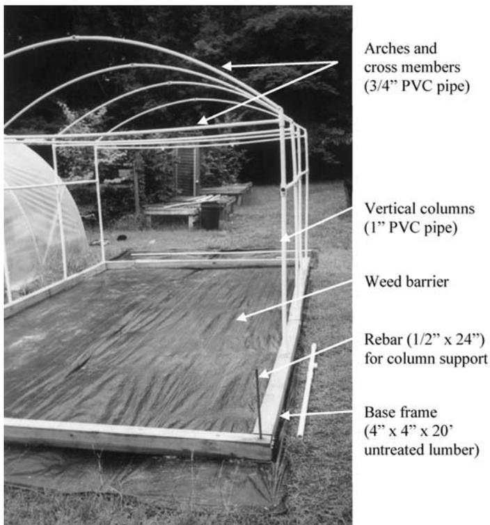
Fig. 1. Structural components of low-cost PVC polyhouse.
