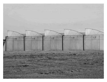
Fig. 2. Greenhouse at the Protected Agriculture Project at the University of Florida. The high roofed structures are passive-ventilated and screened to exclude insect pests.
