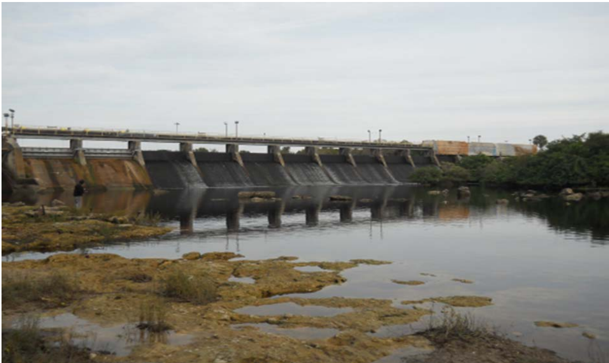
Figure 8. The City of Tampa's dam on the Hillsborough River. Photo by author.
