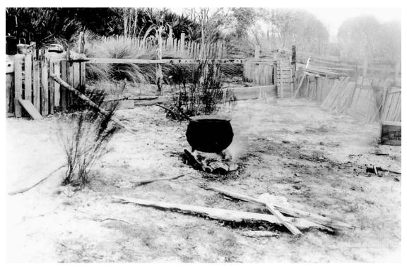
Fig. 6. A 9-gallon iron kettle used by W. W. Yothers to boil oil and water preparatory for emulsification by a bucket pump. Photo by W. W. Yothers, 1910.
