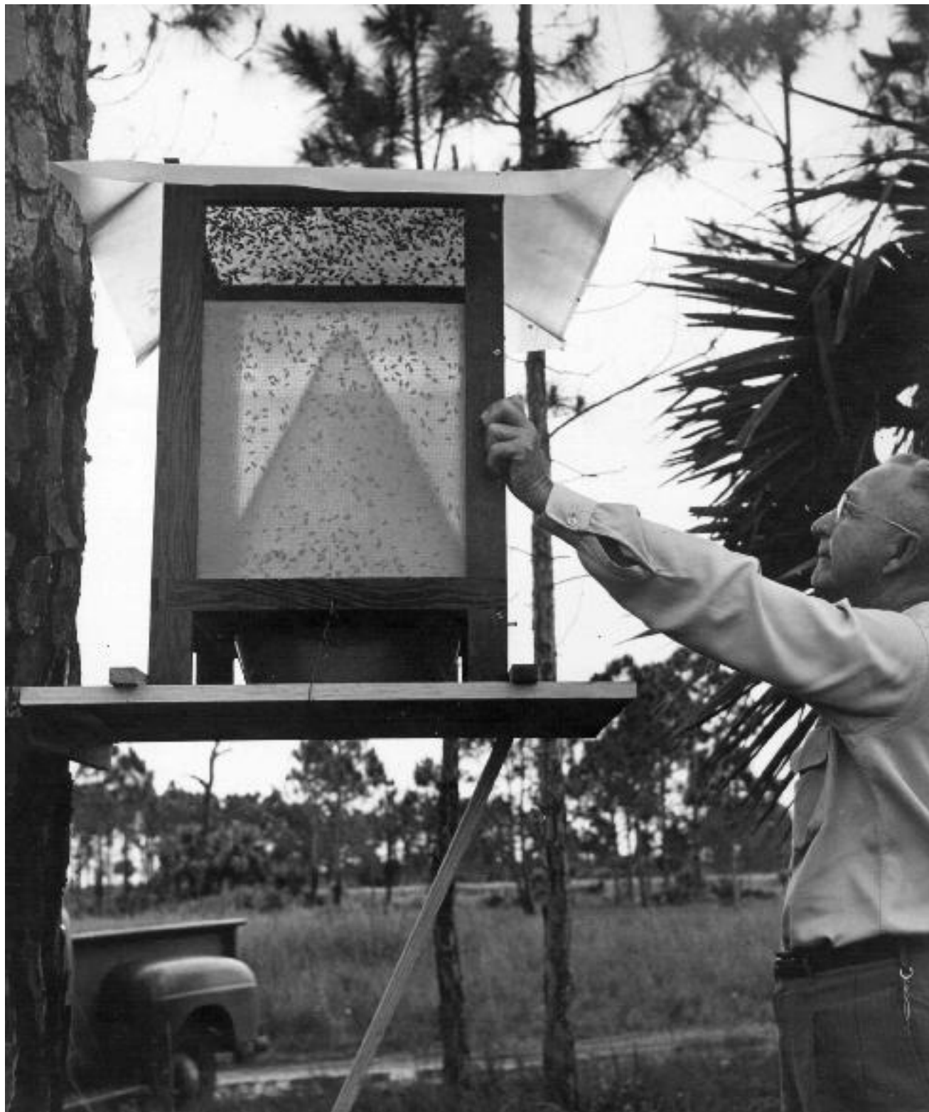
Fig. 21. C.C. Skipper, Survey Specialist, inspecting a liver-baited trap that attracts female screwworm flies along with many other flies including the economically unimportant C. macellaria . The trap was used to study movement of the screwworm, ratios of released flies to native flies, and as an additional measure of control, as used in Broward County. (Author)
