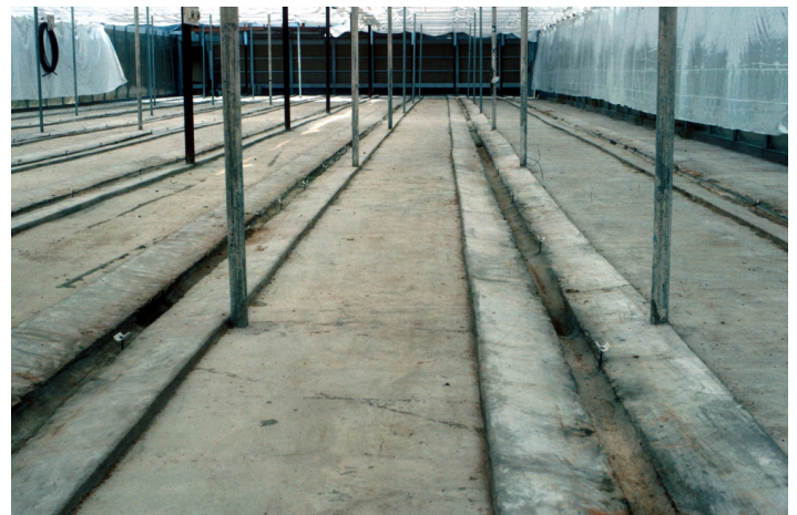
Figure 16. Concrete slanted pads for drainage leachate.
