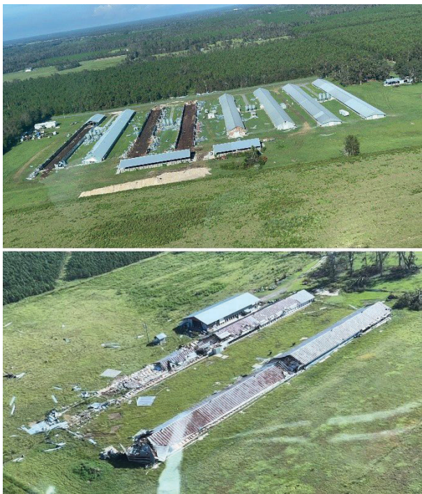
Figure 1. Poultry houses in Suwannee County damaged by Hurricane Idalia.
