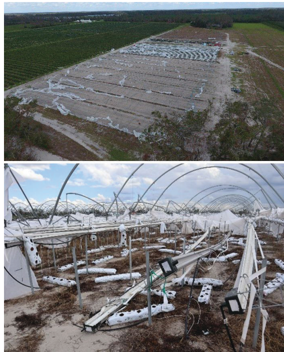
Figure 2. Hoop houses in Lafayette County damaged by Hurricane Idalia.
