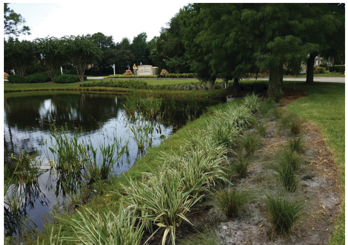
Figure 3. A “no mow” or low maintenance area around community stormwater ponds can protect the ponds from receiving pollutants common in stormwater runoff, such as excess nutrients from yard waste.
