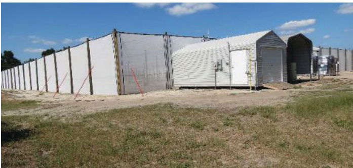
Figure 4. The UF/IFAS CREC CUPS facility near Lake Alfred, Florida.
