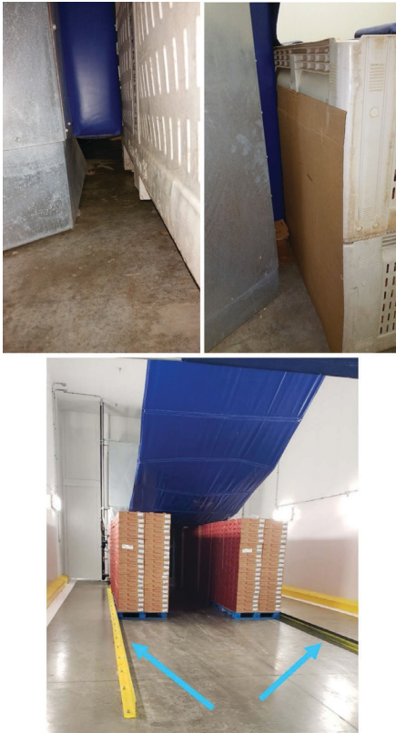
Figure 8-6. Side view at the front of a forced-air cooling tunnel showing: (top left) openings under blue foam pad and at the base of the white adjoining bin; and (top right) these openings blocked with corrugated sheets to improve cooling efficiency. In the bottom image, the fixed angle irons serve to align the pallets as well as block airflow underneath the pallets. Credits: Mark A. Ritenour, UF/IFAS
