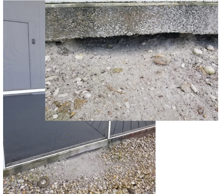
Figure 6. Black spiny-tailed iguana burrow under the foundation of a home on Gasparilla Island. Credits: Sean L. McKnight, UF/IFAS
