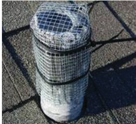
Figure 14. Cover roof vent pipes to keep Cuban treefrogs from invading plumbing systems and showing up in toilets. Credits: Steve A. Johnson, UF/IFAS
