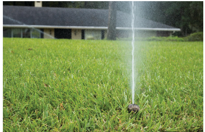
Figure 1. In-ground irrigation at a single-family, detached home in Florida.
