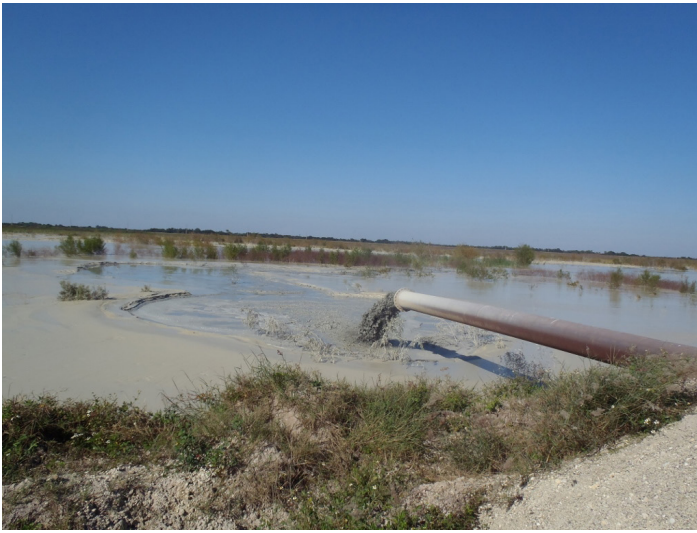
Figure 1. Inlet pipe depositing sand-clay mix. Credits: M. Wilson
