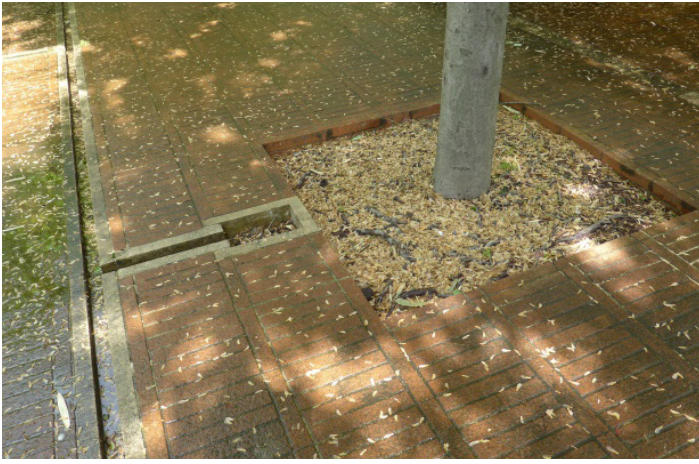
FIGURE 11. Small runnels direct rainwater from the hard surface to the tree wells. (Credit: Gail Hansen)
