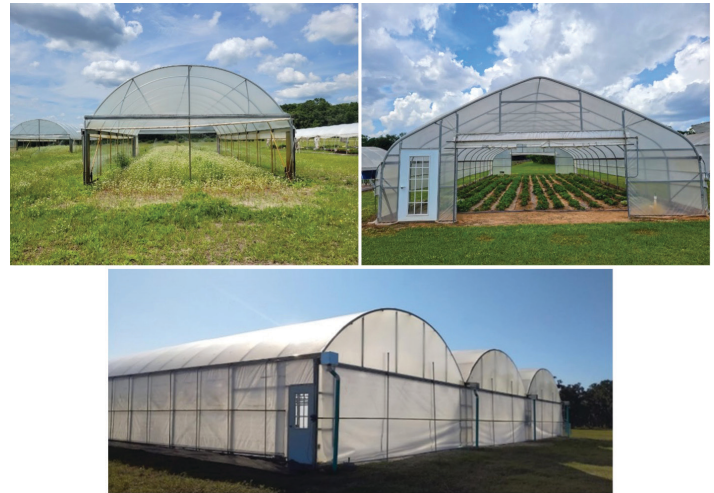
Figure 2. Various styles of high tunnels. Clockwise from the top left: Quonset style, Gothic style, and multi-bay high tunnels.
