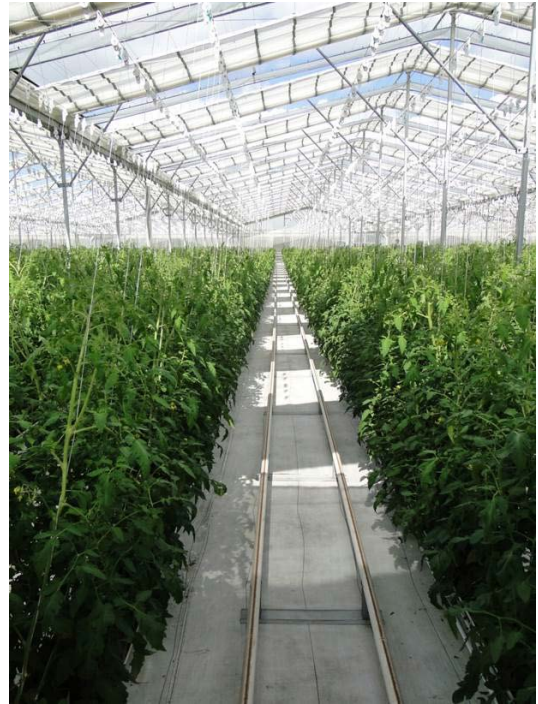
Figure 5. Retractable roof greenhouse with tomato in Ruskin, FL Credits: UF/IFAS
