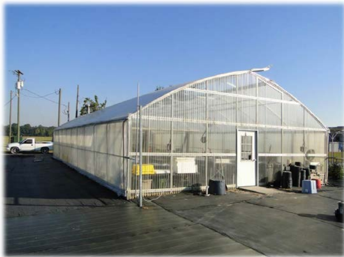
Figure 4. Passively ventilated greenhouse structure Credits: UF/IFAS
