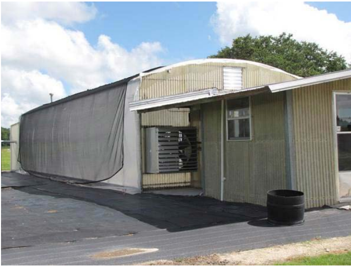
Figure 3. Fan and pad type ventilated greenhouse Credits: UF/IFAS
