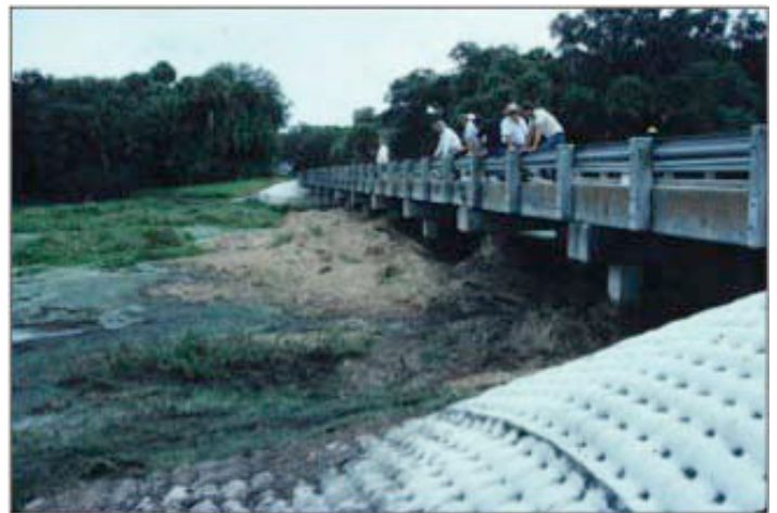
Figure 16. Submersed plants piling up on a bridge in South Florida. Credits: Ken Langeland, UF/IFAS Extension
