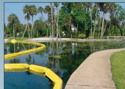
Figure 20. Floating, curtain-style booms keep emergent aquatic vegetation contained. Photograph by UF/IFAS Center for Aquatic and Invasive Plants.
