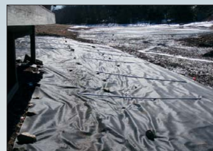
Figure 21. Benthic barrier (Aquascreen®) installed after a drawdown. Photograph by Matthew Vogt, New England Aquatic Services LLC.
