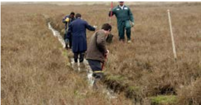
Figure 15. Mosquito control professionals digging a drainage ditch for mosquito source reduction.
