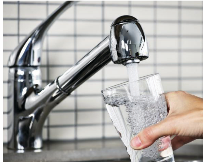
Figure 4. Single-lever faucets are easier to adjust than hot and cold water knobs.
