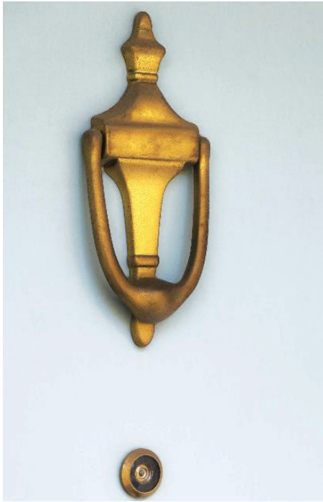
Figure 2. Have a peephole at the right height for you. This will keep you from using a step stool or standing on tiptoes, both of which can be fall hazards.
