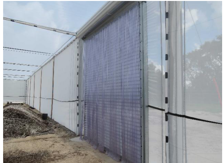
Figure 1. Steel roll-up door with a second plastic strip door, inside the UF/IFAS CREC CUPS.
