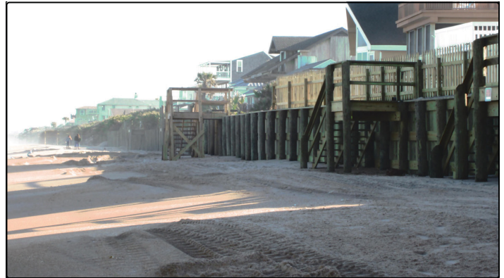
Figure 3. Example of wooden sea walls stretching the length of a Florida beach. Credits: Gary Appelson
