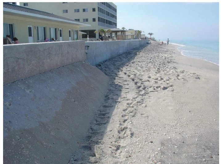
Figure 1. Example of a concrete sea wall where a sea turtle crawled parallel to the wall unable to nest.
