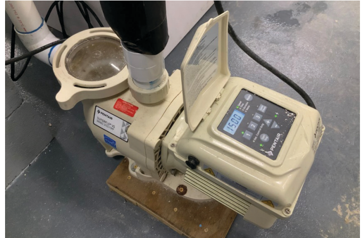
Figure 1. Variable speed pump at the UF/IFAS Tropical Aquaculture Laboratory that provides water flow to one recirculating aquaculture system. This pump uses a DC permanent-magnet motor and DC VSD to control pump speed.
