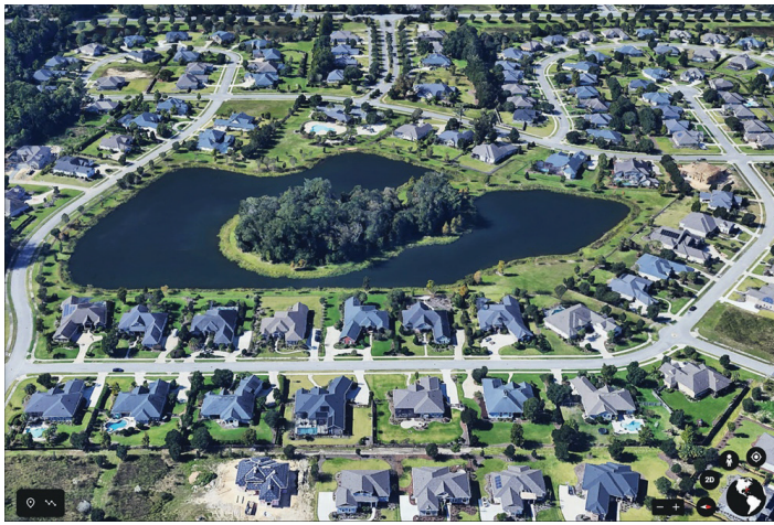
Figure 3. Single-family, detached homes. Credits: Maxar Technologies, U.S. Geological Survey, Google
