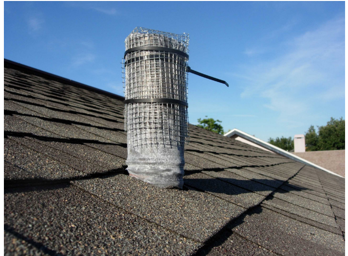
Figure 7. Cover roof vent pipes with hardware cloth to prevent entry into buildings by Cuban treefrogs.
