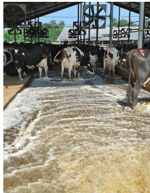
Figure 2. Freestall barn with a flush manure management system in Bowman, SC. Credits: R. Hellmuth
