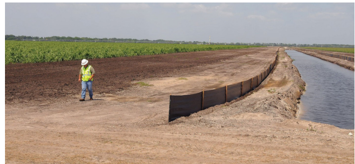
Figure 3. Bare earth buffer and silt fence that were implemented to contain hundred+ acre Napier grass ( Pennisetum purpureum ) planting in Florida, Florida.
