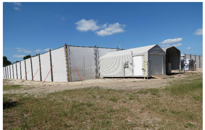
Figure 3. The UF/IFAS CREC CUPS facility near Lake Alfred, FL. Credits: Arnold W. Schumann, UF/IFAS
