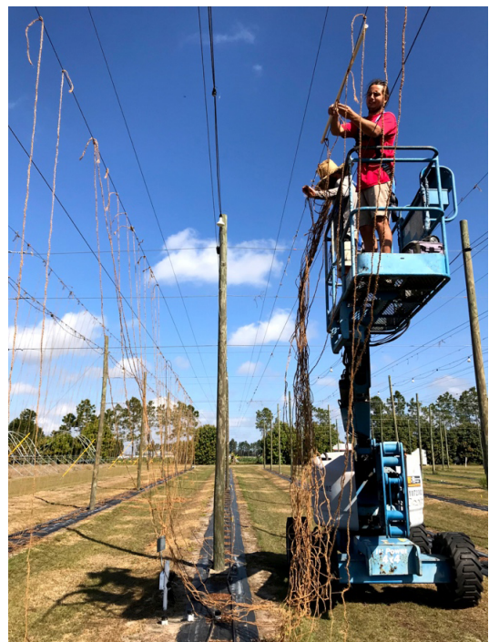
Figure 3. Installing coir twines on a trellis using a scissor lift. Credits: Shinsuke Agehara, UF/IFAS
