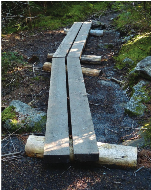
Figure 6. A bog bridge like this can be used to cross a wet area. Credits: David Govatski, Cohos Trail Association
