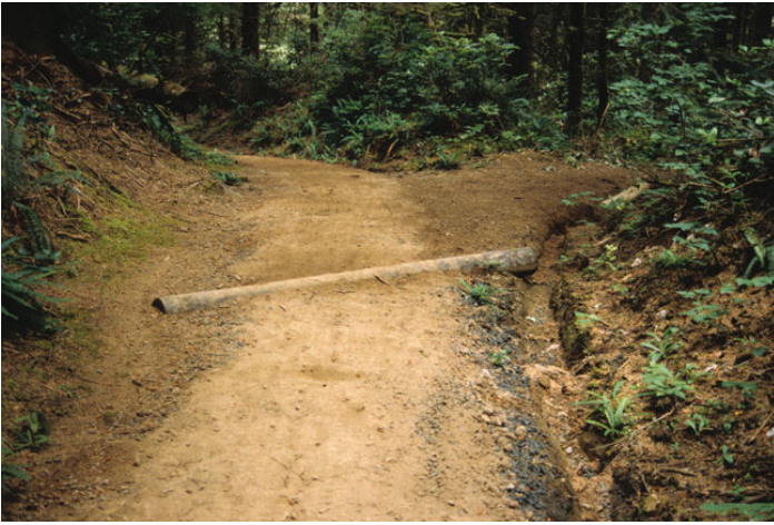
Figure 4. Water bars divert water off the trail without increasing erosion downslope from the trail.
