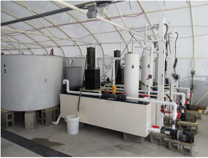
Figure 10. Recirculating system used in the culture of marine ornamental fish.
