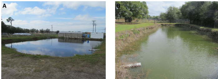
Figure 9. Detention pond (A) and retention pond (B) at a certified aquaculture facility in Hillsborough County. The detention pond discharges through a control structure to a county ditch in the background. The retention pond has no off-site effluent discharge; however, an inflow pipe from an interior ditch is seen in the foreground. The retention pond is underlain by permeable soils and receives little effluent (effluent pipe seen in foreground) from pumped ponds, making this solution feasible.
