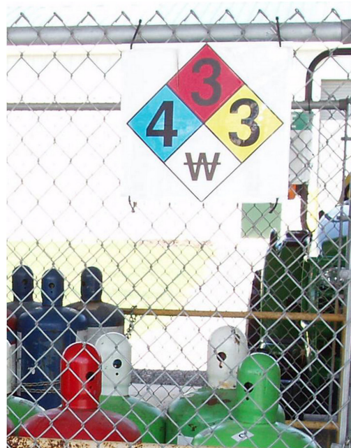
Figure 1. NFPA warning at a fumigant storage site. The strikethrough on the letter “W” in the white diamond alerts firefighters not to use water to put out a fire.
