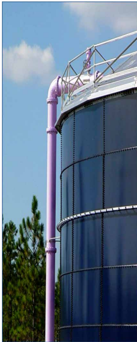
Figure 1. Reclaimed water reuse storage tank. Credits: Shanin Speas, FDEP
