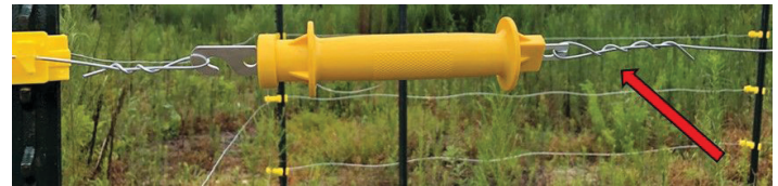
Figure 10. Create enough tension to engage the spring of the handle, then twist the wire onto itself. Credits: K. Post, UF/IFAS
