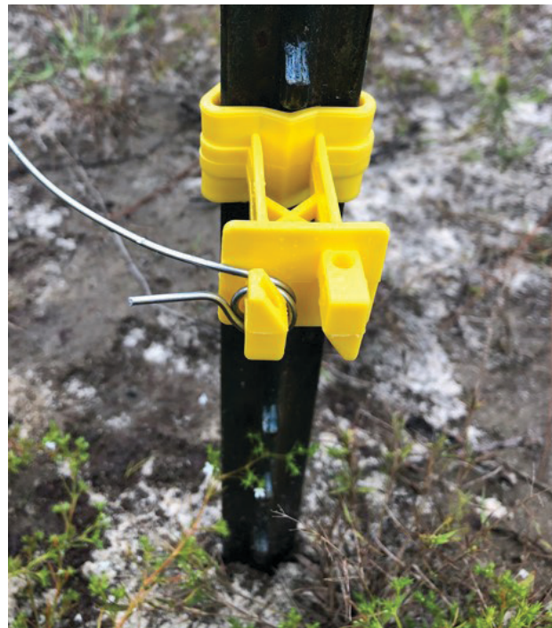
Figure 5. Wrap wire at first insulator. Credits: K. Post, UF/IFAS
