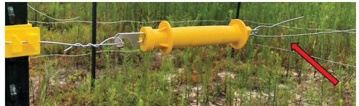
Figure 9. Take the long loose end of wire from that line and run through the spring end of the handle. Credits: K. Post, UF/IFAS
