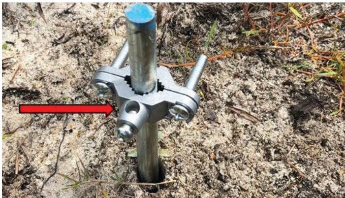
Figure 13. Clamp attached to grounding rod. Arrow indicates where ground wire should be inserted into clamp. Credits: K. Post, UF/IFAS
