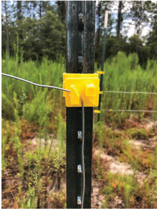
Figure 6. Run wire straight up to next level of insulators. Credits: K. Post, UF/IFAS
