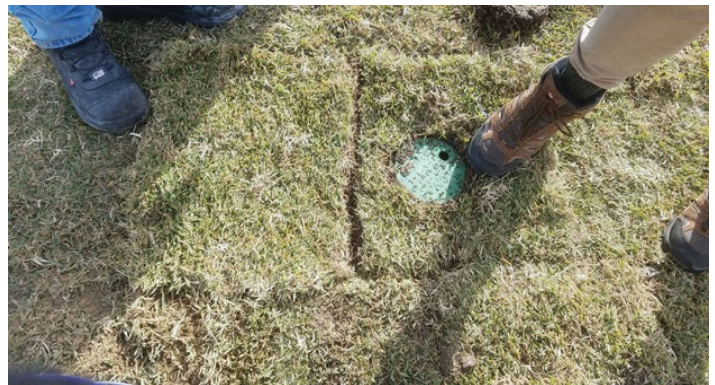
Figure 10. The turfgrass removed before installation was replaced over the lysimeter. An area was cut out of the sod to access the tube housing. Credits: Jovana Radovanovic, UF/IFAS
