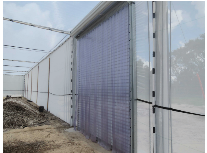
Figure 1. Steel roll-up door with a second plastic strip door, inside the UF/IFAS CREC CUPS. Credits: UF/IFAS
