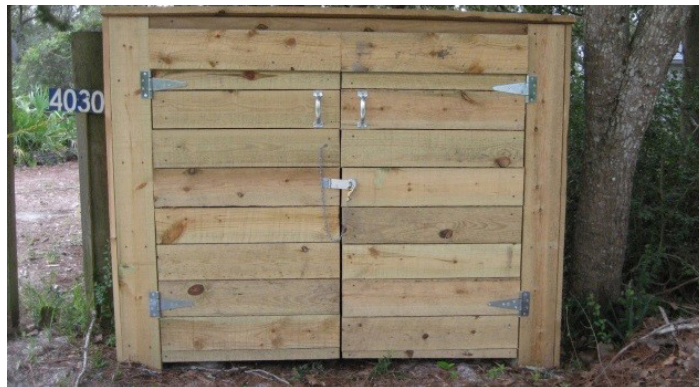
Figure 3. A bear-resistant caddy designed to secure garbage cans before pick-up. Credits: FWC
