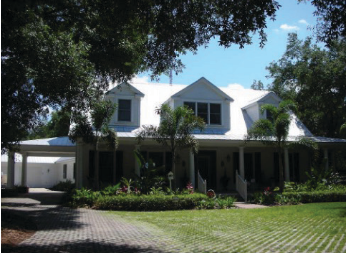
Figure 27. Pervious pavement. Credit: UF/IFAS Florida-Friendly Landscaping™ Program
