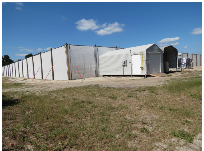
Figure 3. The UF/IFAS CREC CUPS facility near Lake Alfred, FL. Credits: Arnold W. Schumann, UF/IFAS
