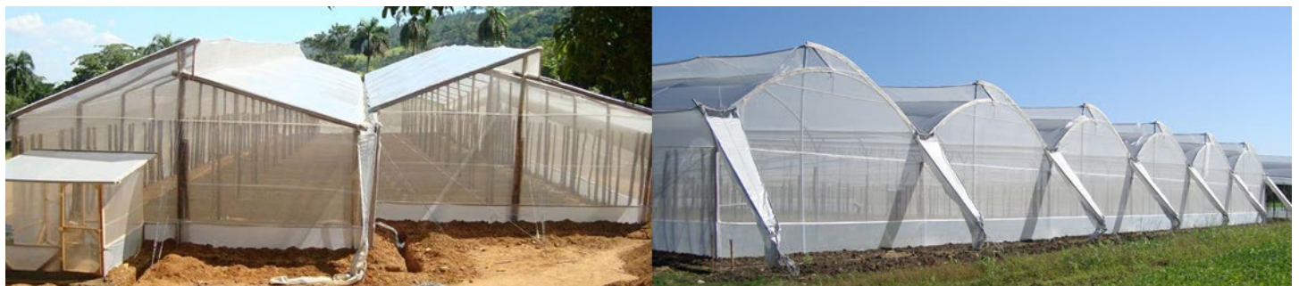
Figure 3. Multi-chapel (left) and semi-cylindrical (right) greenhouse units with passive ventilation on roofs Credits: B.M. Santos
