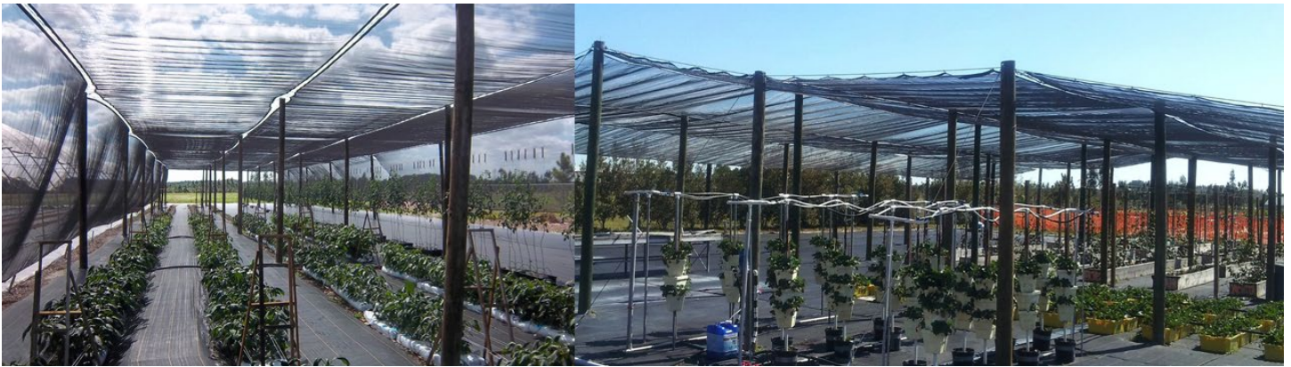
Figure 2. Shade houses for vegetable and small fruit production Credits: B. M. Santos
