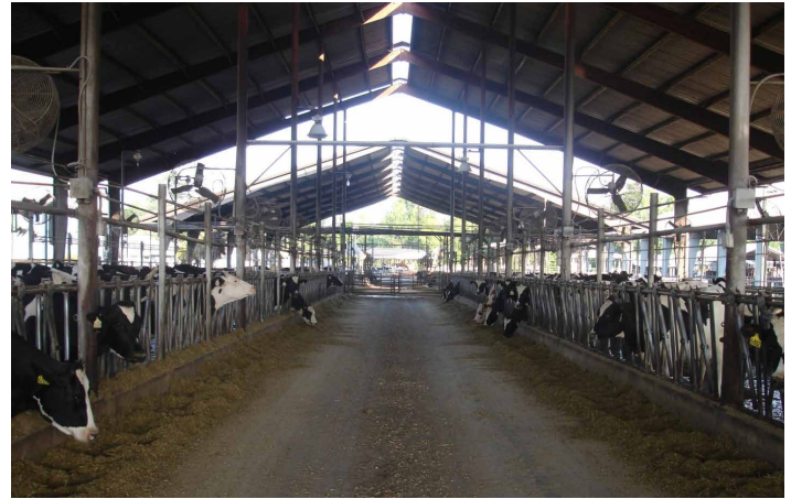
Figure 2. Picture of the barn on the south side. Credits: K. Galvão
